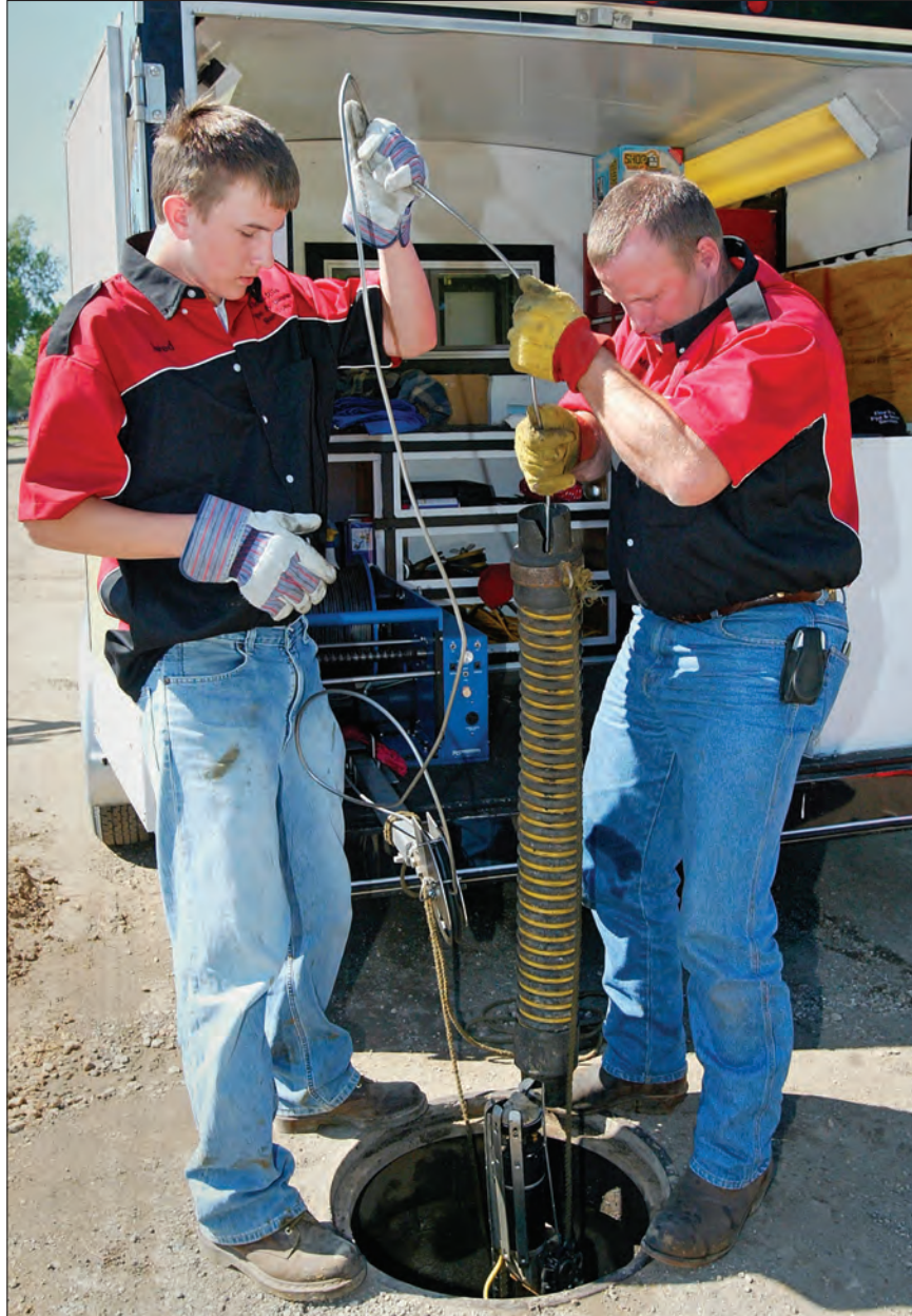
Mike Happel (right) and Jared Happel remove a camera from a manhole after an inspection.
